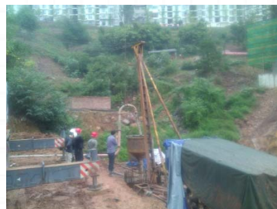
site ready to concreting
