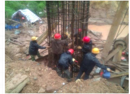
jointing rebar sections
