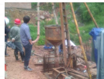
concreting to 2m dia. pile
