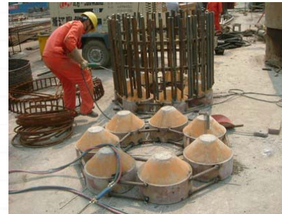
fabrication of Y-jacks at site
