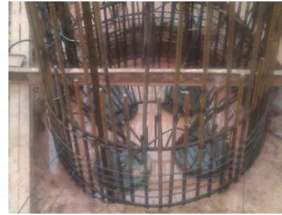
Y-jacks & cables in bore-hole
