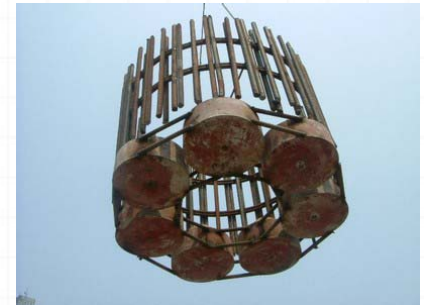
Y-jacks at top rebar section
