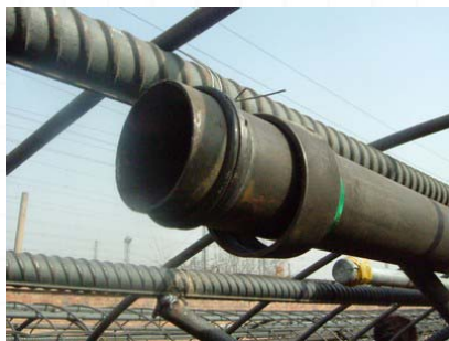
5cm pipe for grouting
